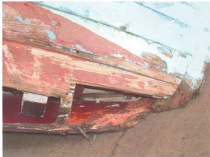
Figure 3. Foot of bow, with scarf joint in stem, base of Samson post, and missing keel
