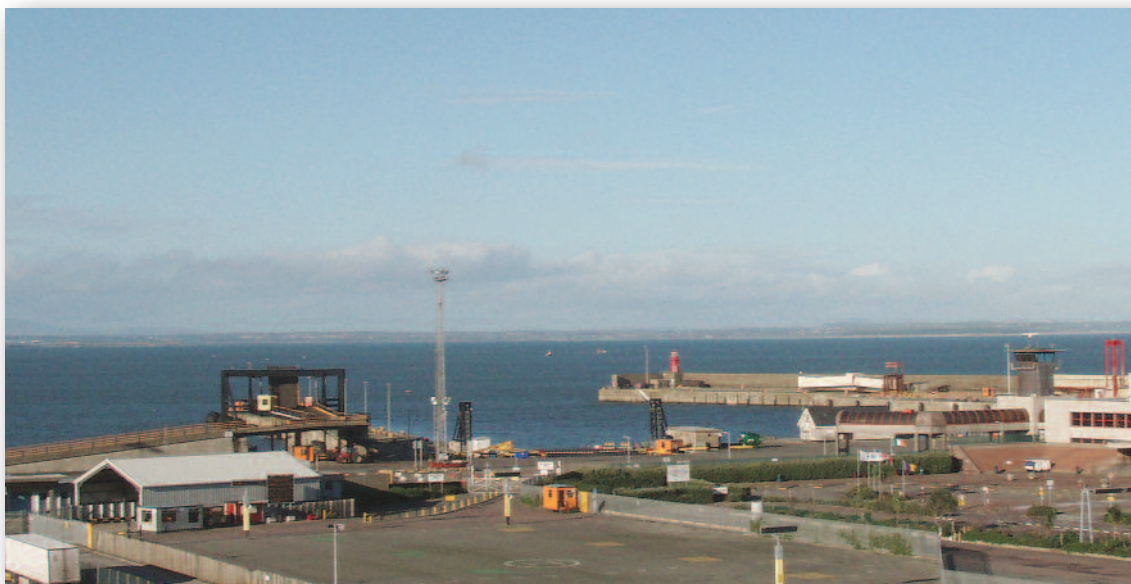
Rosslare Harbour, Berth 2 to left and Berth 3 to right. CCTV mounted on control tower to right.
