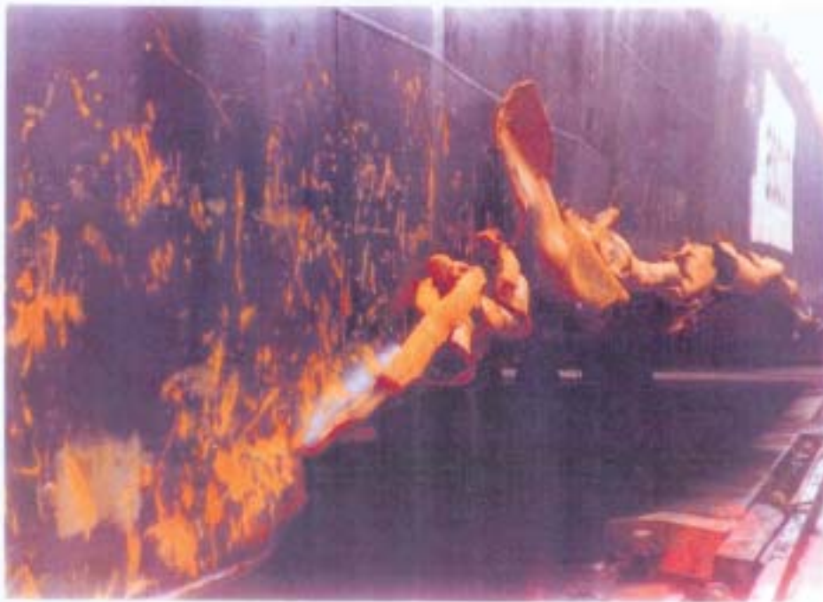
PHOTOGRAPH NO. 2 SIDE SHELL
