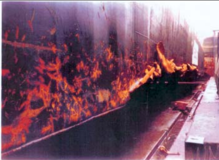
PHOTOGRAPH NO. 1 SIDE SHELL
