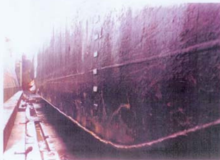
PHOTOGRAPH NO. 4 SIDE SHELL
