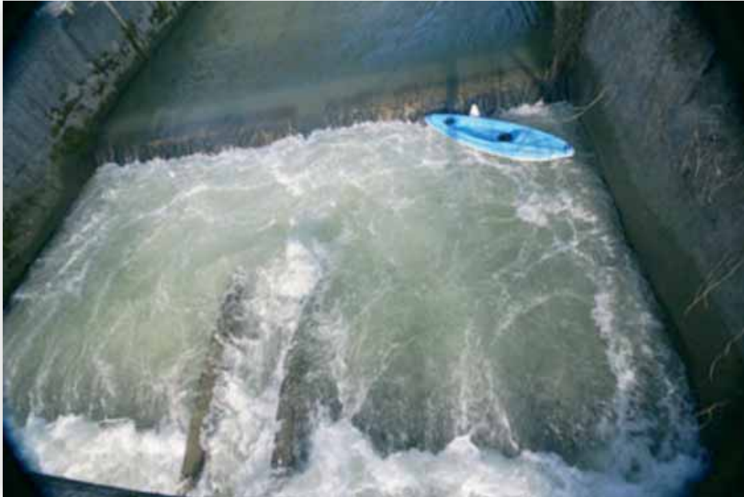
Note that the Bic Sports Kayak sit-on type Kayak is lodged firmly in the weir back flow after twelve hours.
