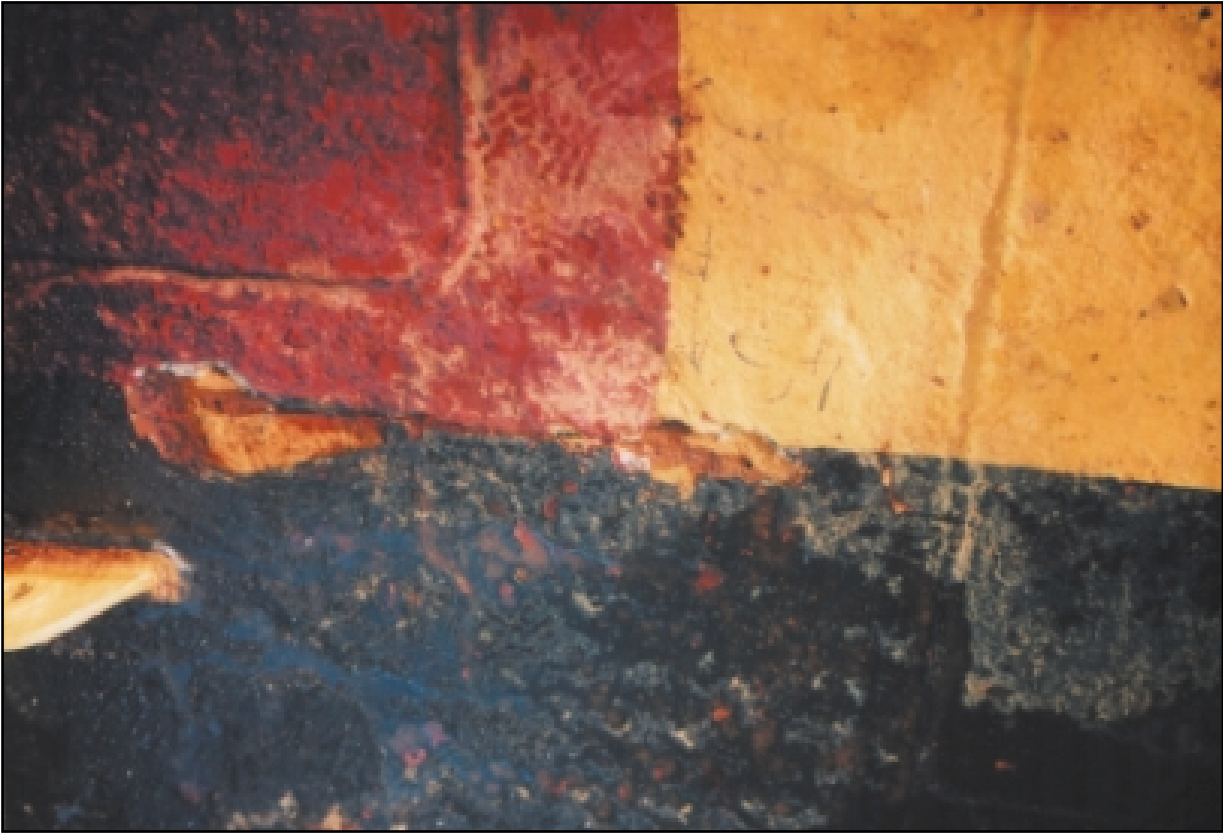
Figure 7.1.8 Crack at frame 59 starboard side length approx. 0.8 m
