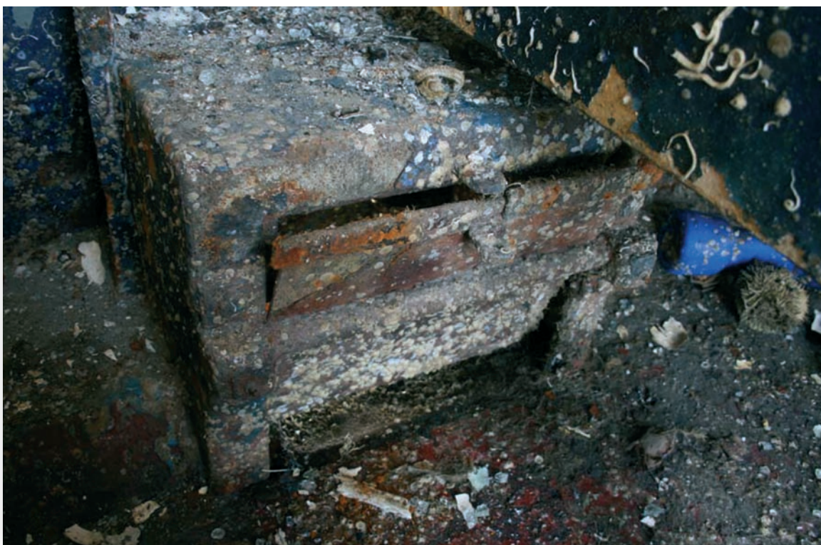
Photograph 9 - Freeing Port D (Port) viewed from inside (showing siezed hinged cover).
