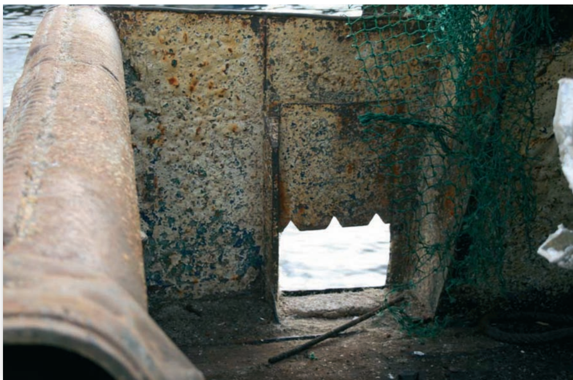
Photograph 7 - Freeing Port D (Port) viewed from outside.
