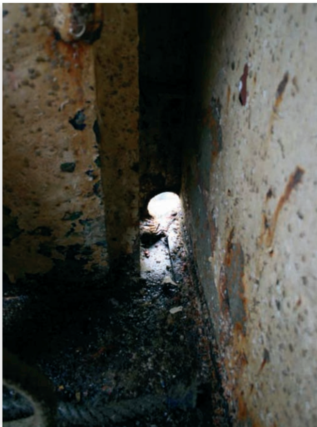
Photograph 10 - Freeing Port E (Port) viewed from inside.
