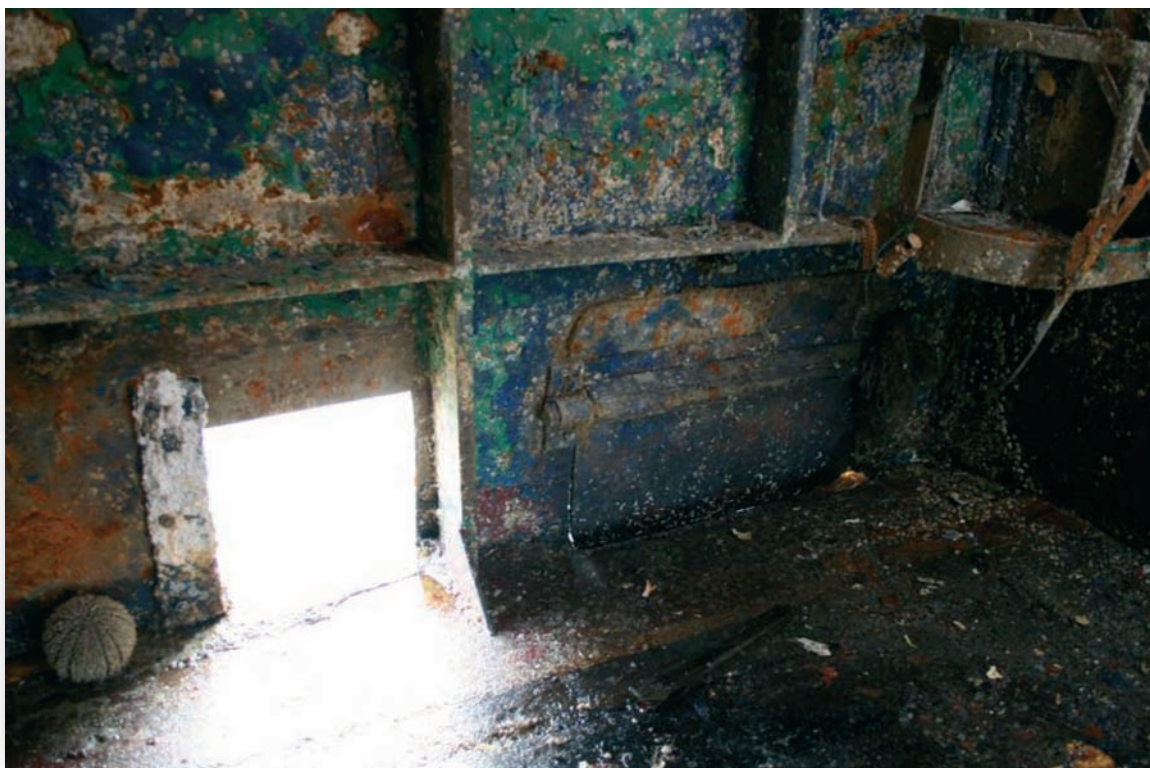
Photograph 4 - Freeing Ports B and C (Port) viewed from inside.
