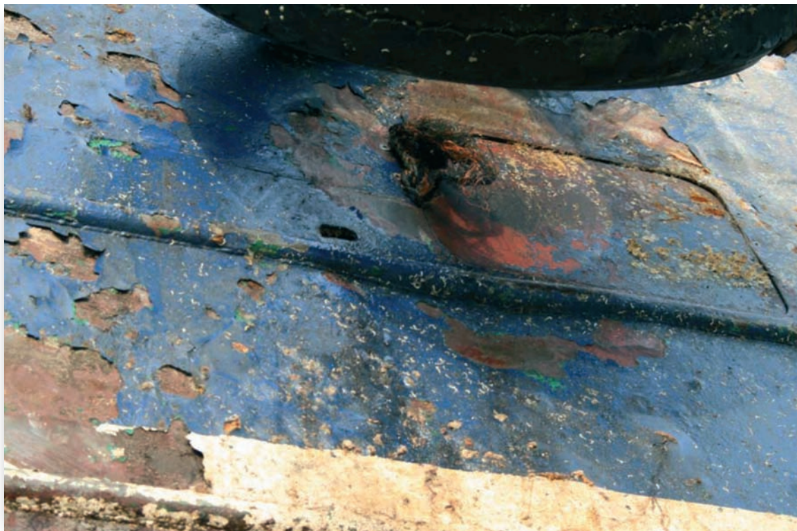
Photograph 6 - Freeing Port C (Port) and 'small hole' viewed from inside.
