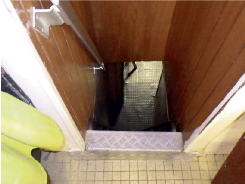
Photograph No. 3 - Looking down the stairwell from main deck.
