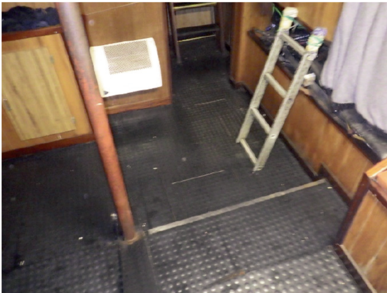
Photograph No. 8 - Looking at deck forward starboard.
