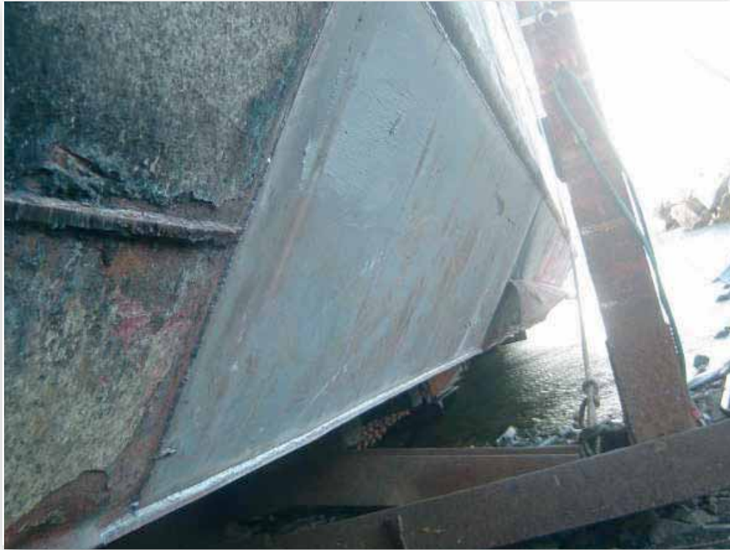
Appendix 8.4 Photograph showing new plate after repair.
