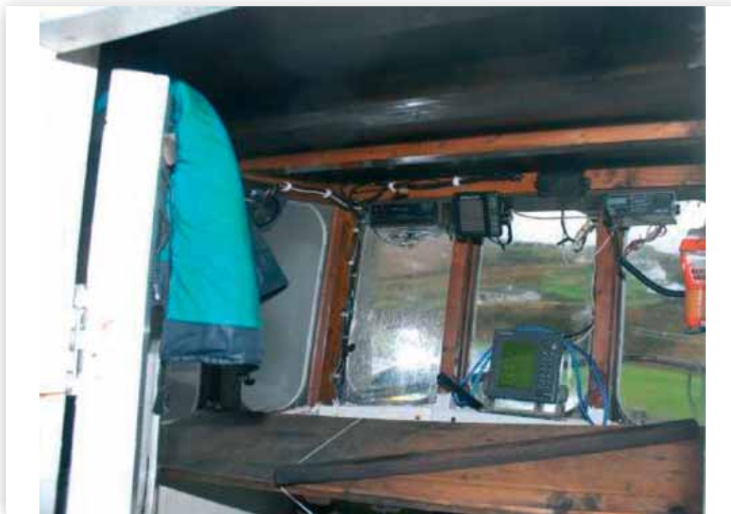
a) Photographs of Wheelhouse internally after salvage.
