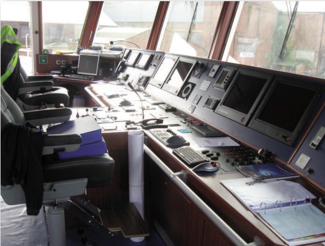
Appendix 7.3 Photograph of control console section being used by Master.
