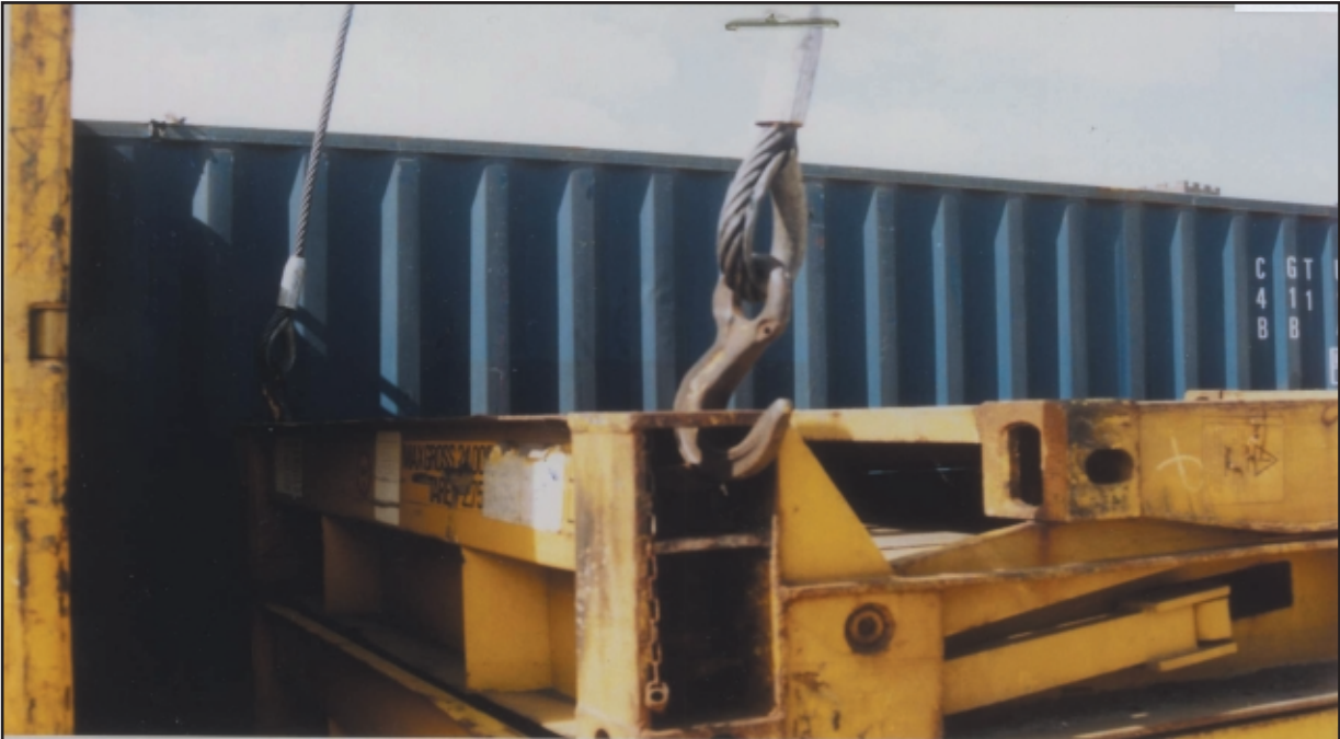
Photograph “d” shows the hooks rigged to the top flatback in the correct manner that would avoid the inboard hook(s) being jammed against the inboard 40 foot container “B”. Refer to paragraph 5.15.6.
