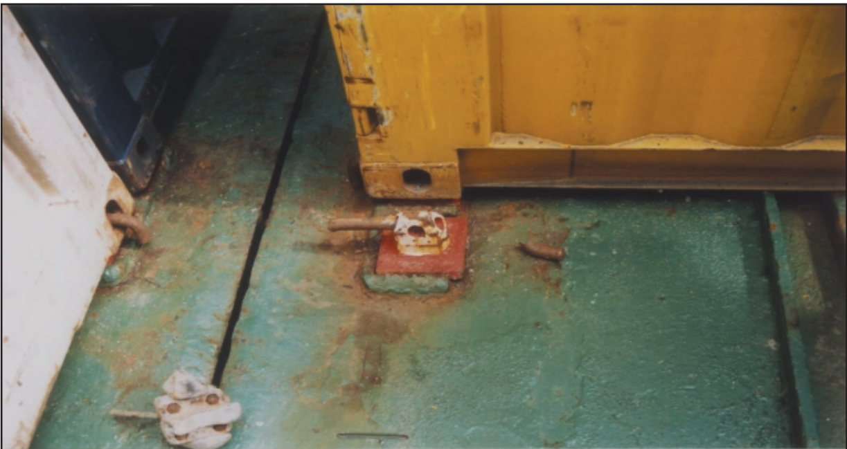
Photograph “e” Shows the method of securing the first tier containers to the hatch lid as described in paragraph 5.15.2. A sheared section of the locking bar is lying to the right of the shoe and a twistlock can be seen in the front and to the left of the photograph.
