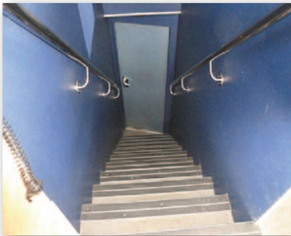
View of Stairwell from Top
