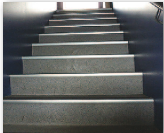
View of Stairwell from Bottom
