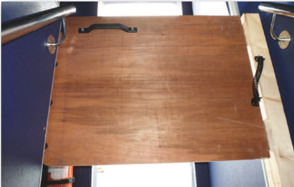
Spring Loaded Gate Subsequently Fitted at Top of Stairs, Preventing Accidental Stepping onto Stairs.
