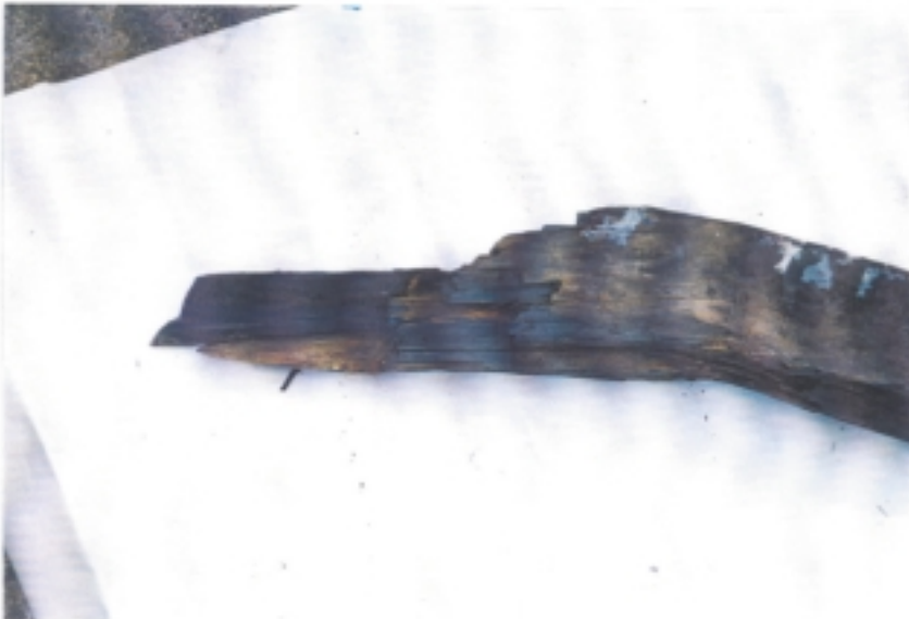
Figure 4. Frame 2. Rust on pre-existing splits, black surfaces freshly broken.
