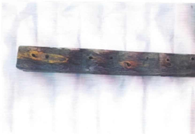
Figure 2, Frame 1. Erosion and softening of wood at fastenings.
