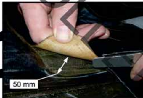
Corners with lifting patch FIGURE 6
