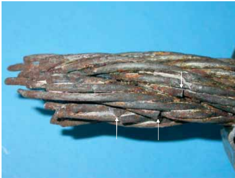
Figure 32: Port Side Fixed End sample, showing sites of transverse fatigue like fractures of individual wires.
