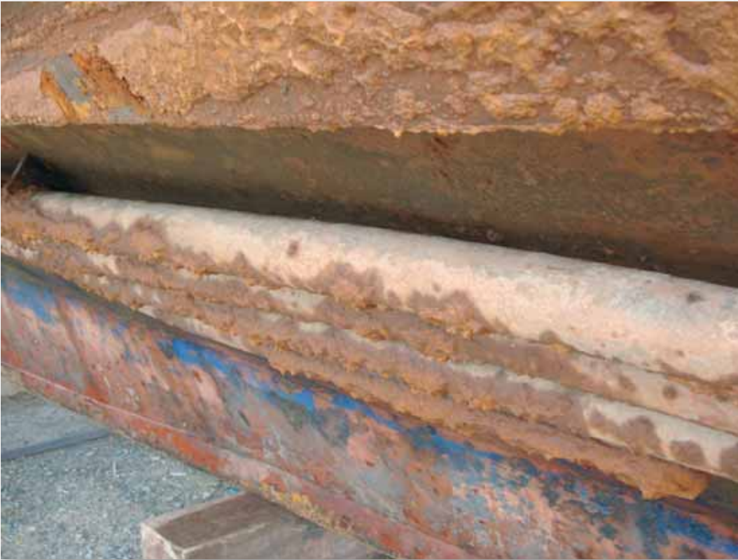
Appendix 3.3 Photo 6 showing keel cooler.
