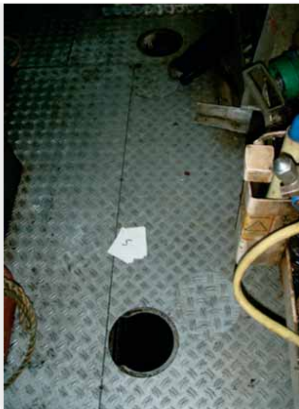
(a) Access to the port & starboard valves for VIVER suction.
