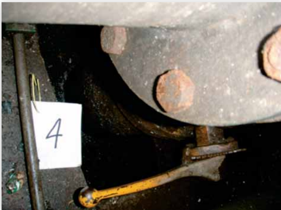
(b) VIVER suction valve showing inlet pipe to hull.
