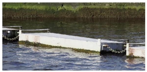
Figure 14: Example of the safety boom in place above the weir.
