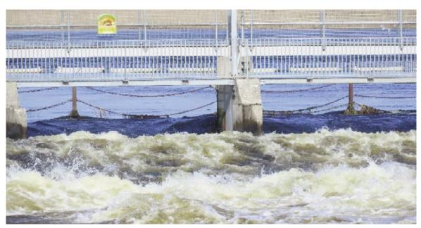
Figure 11: The chain protection, immediately above the Salmon Weir. Viewed from downstream.
