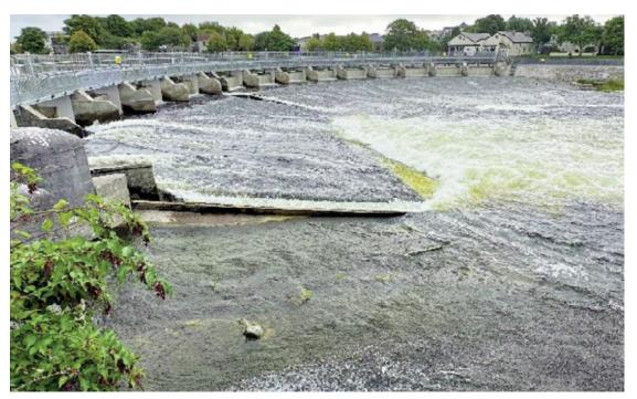
Figure 7: The Salmon Weir during summer flow conditions (in August 2023), when only two of the 16 sluice gates are open.
