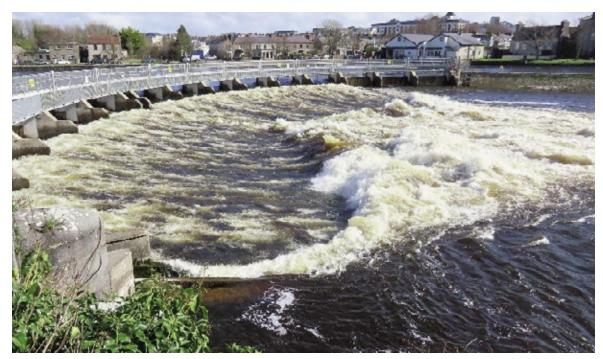
Figure 6: The Salmon Weir during winter flow conditions (in March 2023), when all 16 sluice gates are open.
