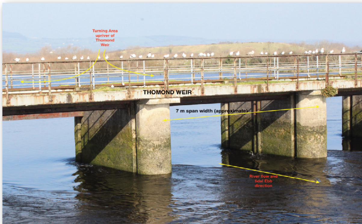
Thomond Weir - Support Spans.
