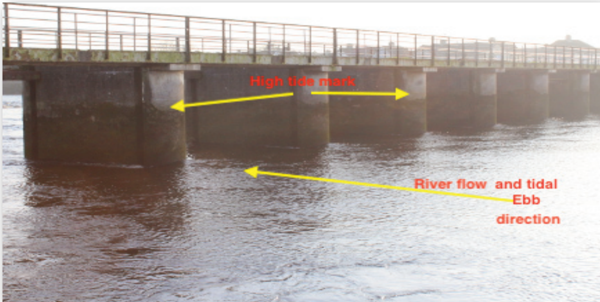
Thomond Weir - Upstream View (north side).
