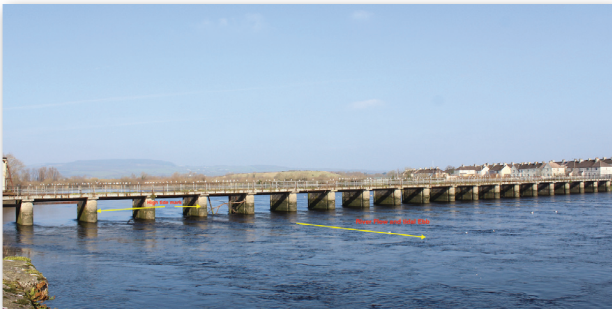
Thomond Weir - Downstream View (south side).
