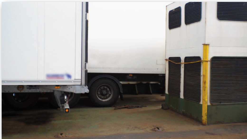
Photograph No. 3: Ventilator shaft.
