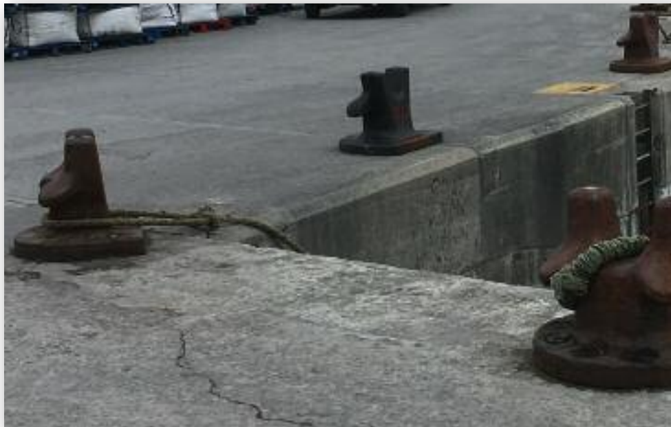
Photograph No. 3: Staghorn Bollards.
