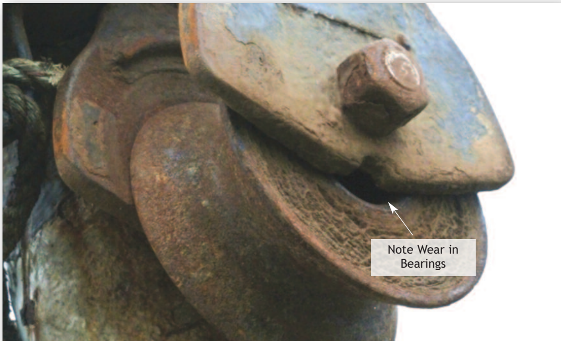
Photograph No. 7: Close-up of Head Block
