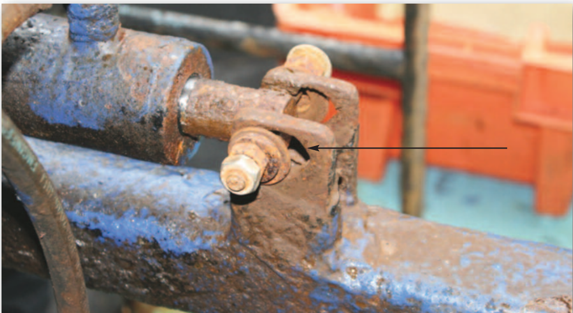
Photograph No. 10: Wear in Winch Guiding on Gear Securing Arrangement
