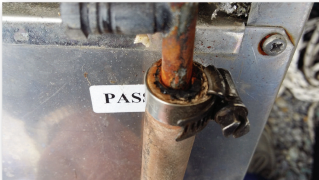
Photograph No.4 - Gas hose refitted to cooker hose tail.
