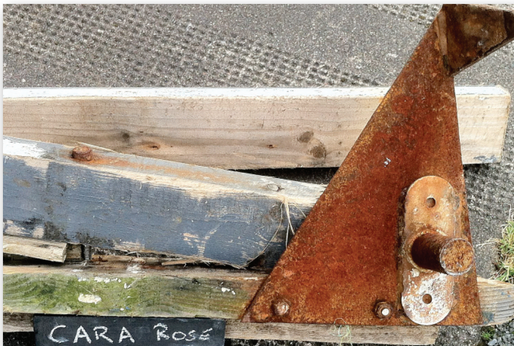
Photograph No. 9: Lower Socket for pot hauler secured to deck beam.
