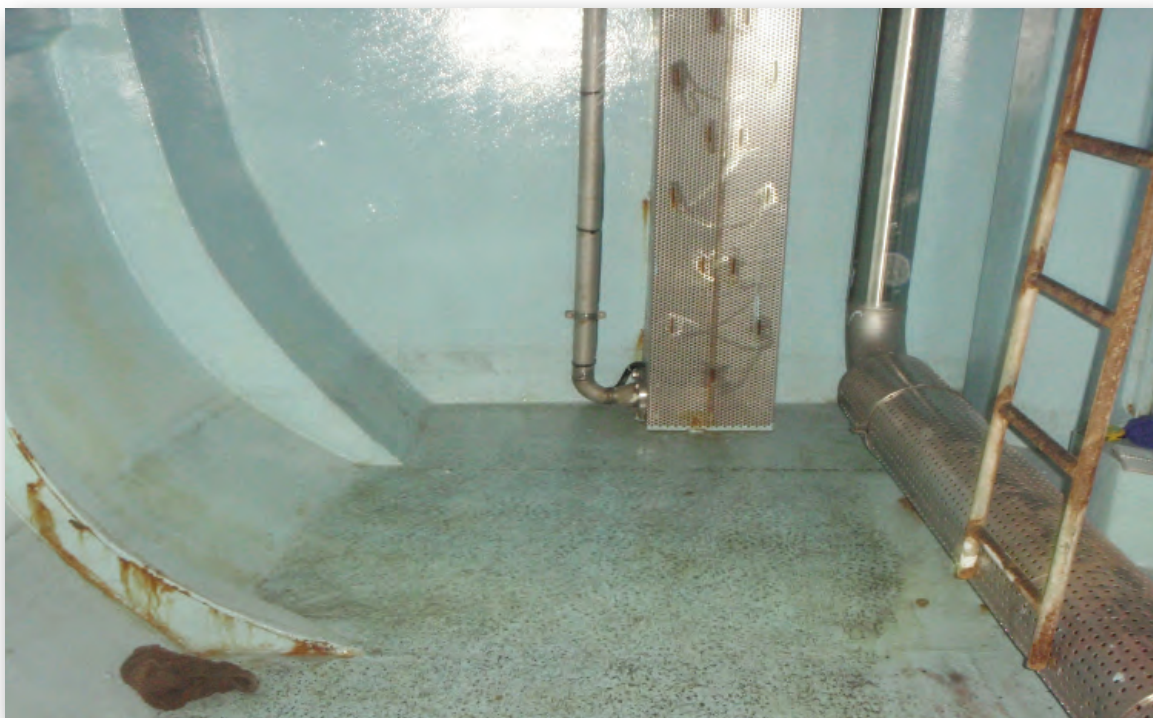
Photograph No. 2: Port Side Refrigerated Sea Water Tank.
