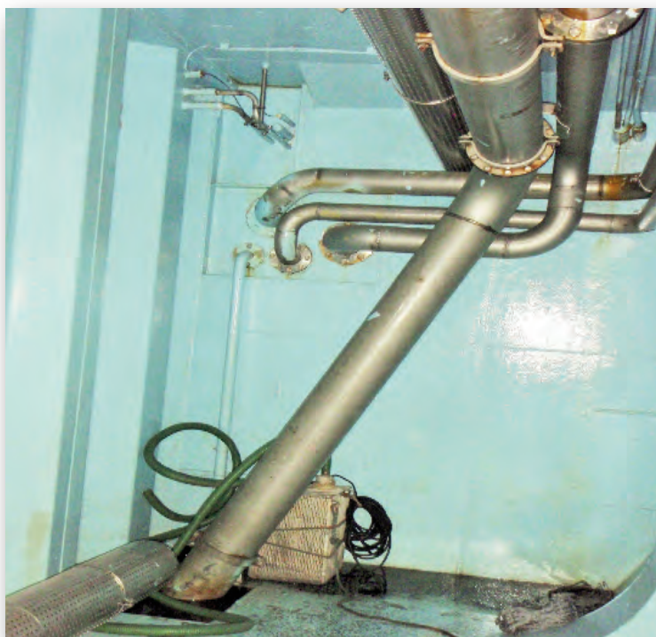
Photograph No. 3: Port Side Refrigerated Sea Water Tank.
