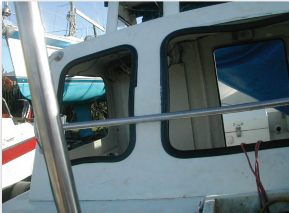
Photograph 3 - Damage to forward facing windows suffered by “ Jillian ” during the incident.
