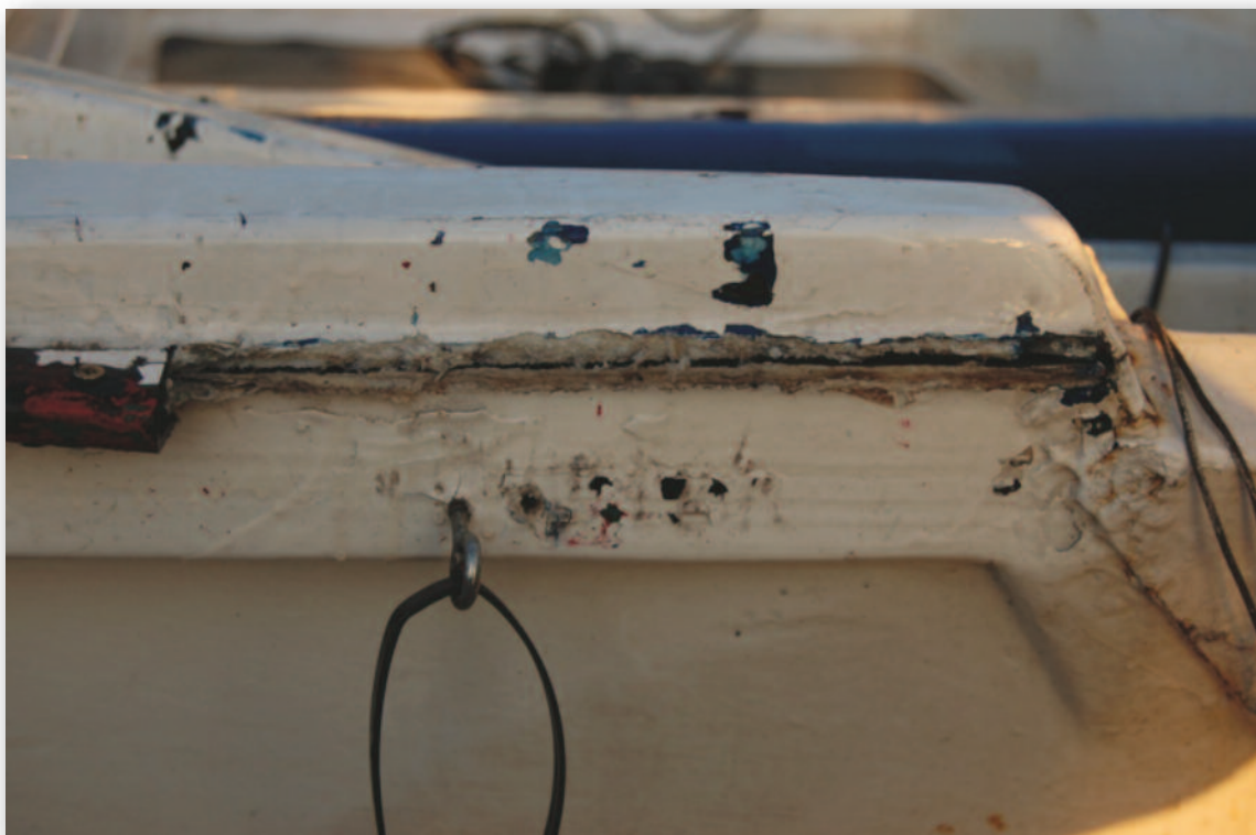
Photograph No. 4 - Showing the damage to the hull deck joint
