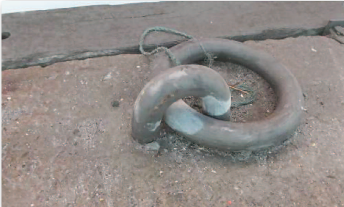
Photograph No. 9 - Similar ring showing how it is set into apron
