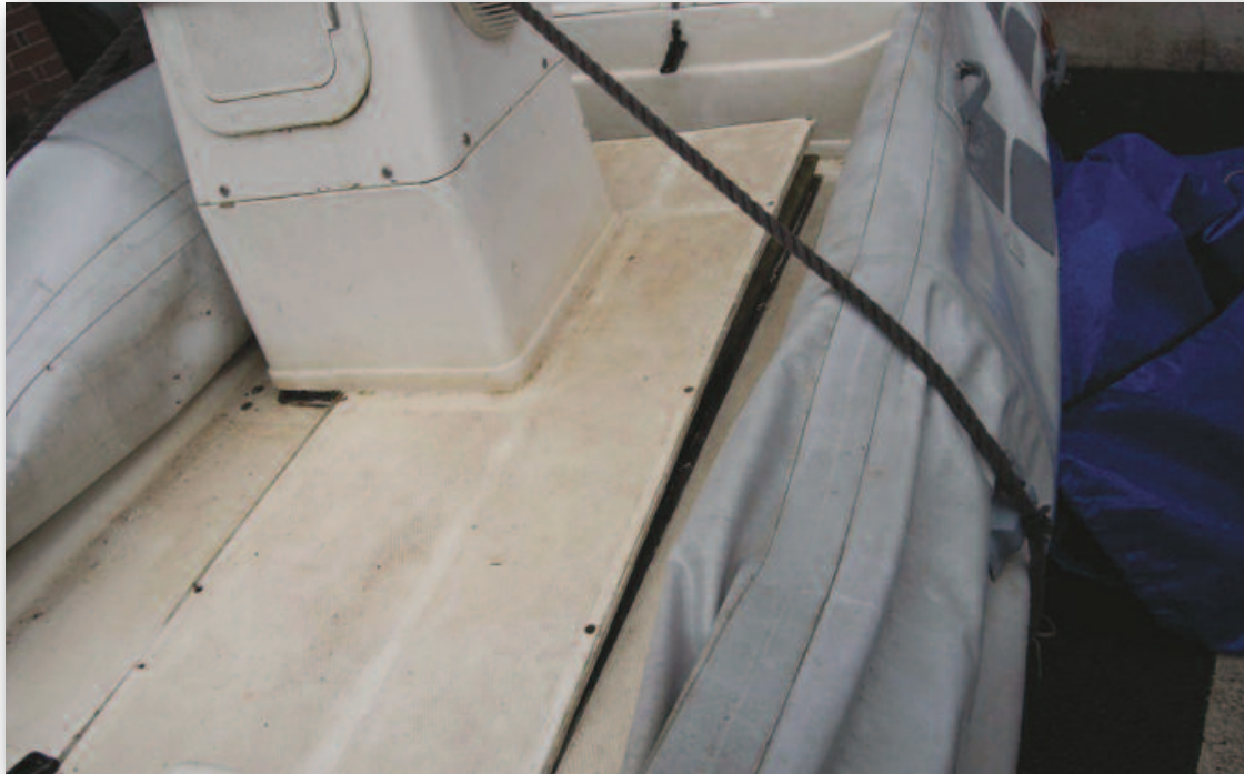
Photograph No. 5: Console and the deck lifted to reveal the inboard fuel tank beneath
