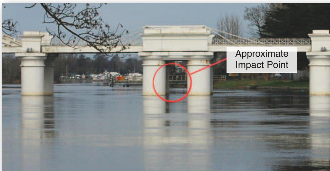
Appendix 7.3 Photograph of the Athlone Railway Bridge.
