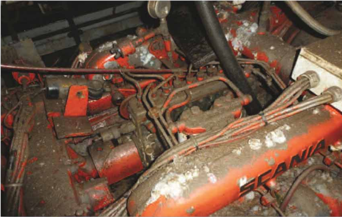
Photograph No.17 - Top of main engine fuel lines split to obtain samples
