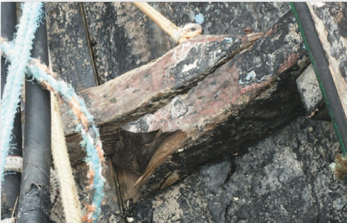
Photograph No. 6 - Typical Internal Timbers of Vessel
